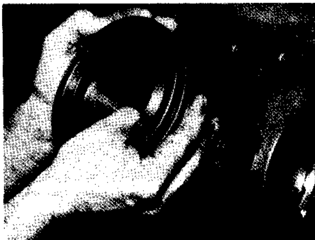
Figure 7 — Installing Cylinder Liner
