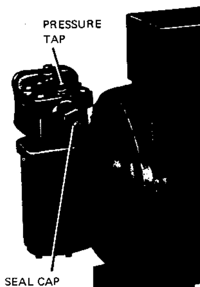
FIG. 3 — SUCTION STOP VALVE
